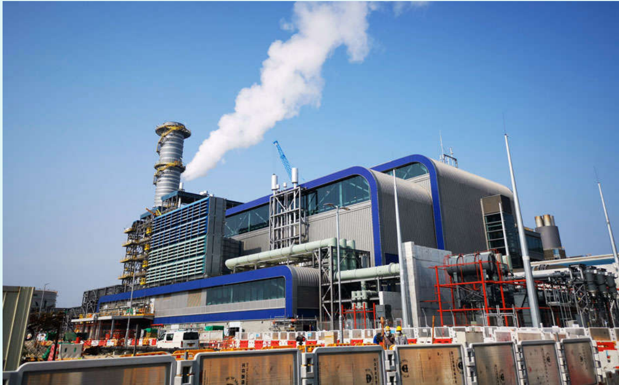
The new CCGT unit at Black Point power station is expected to be in operation in 2020.
