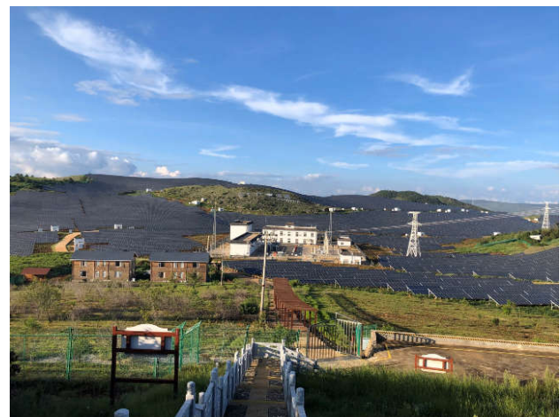
The Xicun Solar Power Station integrates the farming of honeysuckle plants into its operations.
