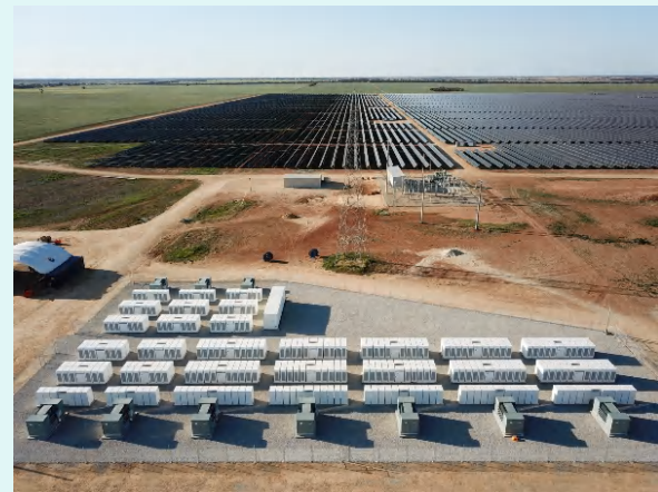
The large battery at Gannawarra, underpinned by EnergyAustralia, is an example of the changing technologies shaping the energy system.
