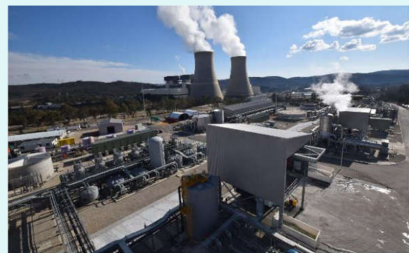
The Springvale Water Treatment Plant built next to the Mount Piper Power Station.
