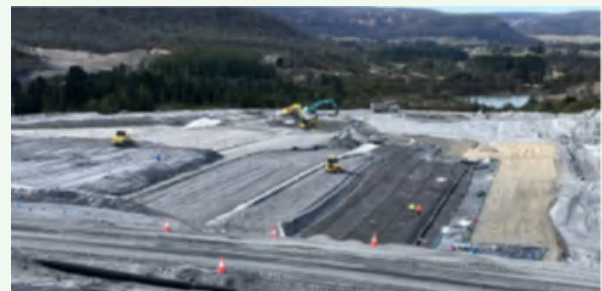
Installation of the Leachate Barrier Management System at the Mount Piper Power Station
