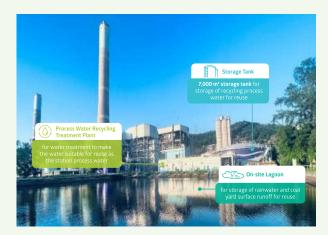
The process water recycling treatment system was installed to treat process water and enable recycling in CPPS following the surrender of the Tsang Tsui Ash Lagoon (TTAL) to the government. Wastewater treated by this system will be suitable for reuse at the plant. In addition, with this new system, the water management process at CPPS no longer depends on the TTAL. The land will be released for alternative land for the benefit of the community.
