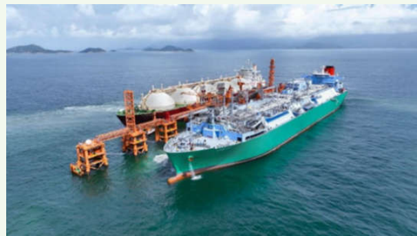
The Hong Kong Offshore Liquefied Natural Gas (LNG) Terminal.
