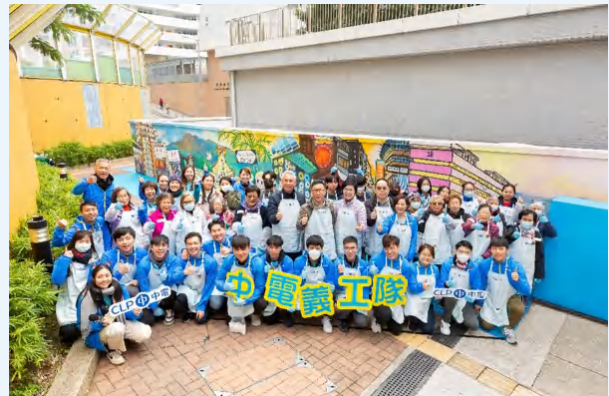
Residents of all ages teamed up to beautify the substation in Shek Kip Mei with colourful messages about local heritage and the importance of low-carbon lifestyle.
