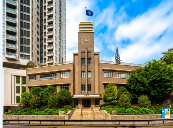
CLP Pulse, a unique cultural hub housed in CLP’s renovated clock tower building, promotes heritage, culture and green education for the benefit of the Hong Kong community.
