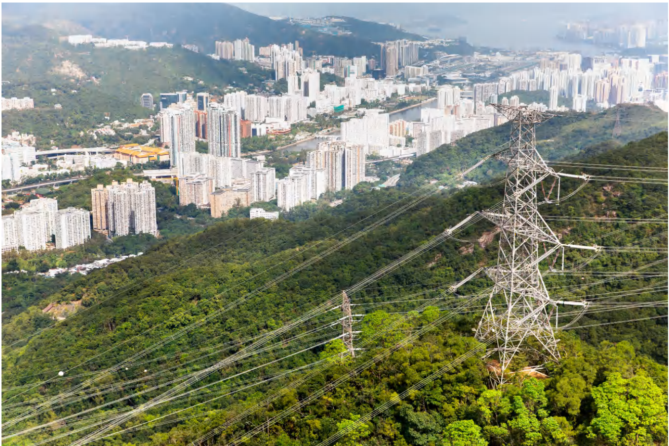
Maintaining proper Health, Safety and Environment management practices for transmission towers is important to keep the general public safe.
