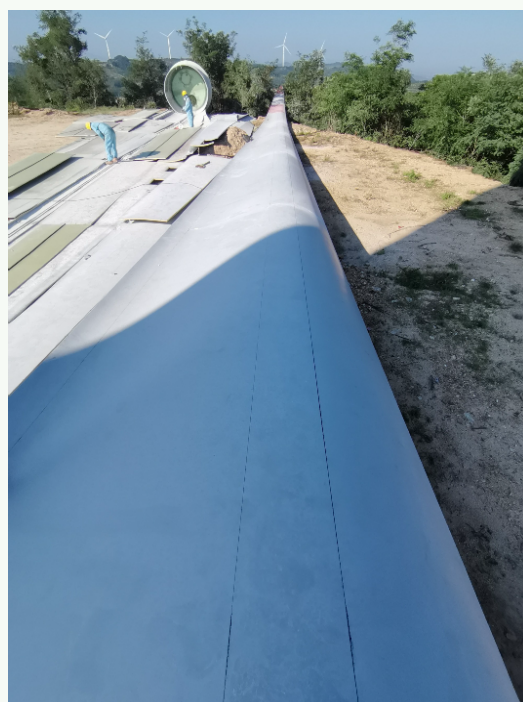
Process of cutting and shredding to recover and repurpose retired wind turbine blades
