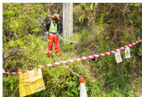
A CLP Power worker carried out pole cleaning, removing nearby weeds and tree branches to minimise their impact on power facilities in the case of a hill fire.
