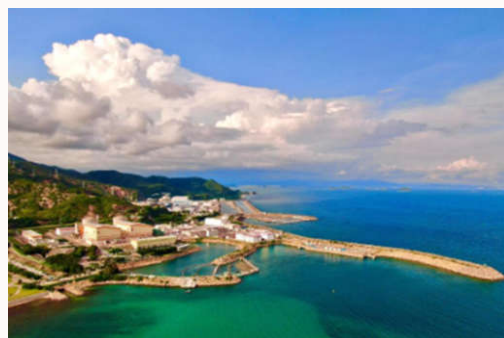
Daya Bay Nuclear Power Station was commissioned in 1994 and has supplied Hong Kong with safe, stable and non-carbon emitting nuclear power for over 30 years, meeting a quarter of Hong Kong's electricity demand.
